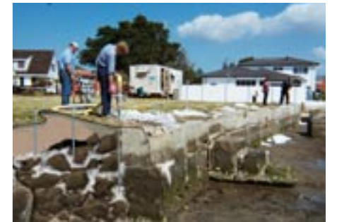
'Spearing' behind seawalls to replace lost 'fines'. Benefil encapsulates rocks and fills voids
