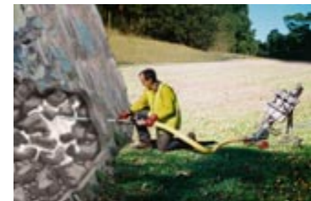
Voids filled and rocks encapsulated
