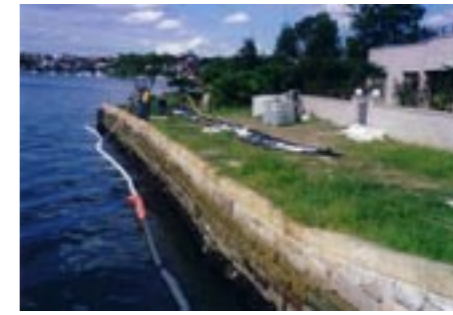
'Spearing' behind seawalls to replace lost 'fines'. Benefil encapsulates rocks and fills voids
