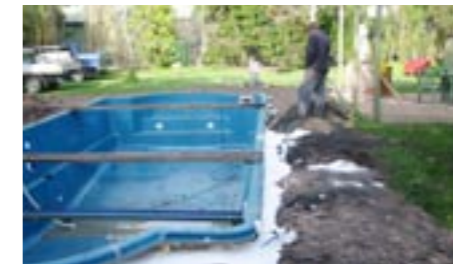
New fibreglass pools may be filled with water immediately or as soon as convenient
