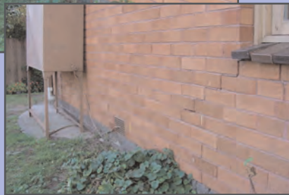
These sets of 'Before' and 'After' photos show how cracks in walls and gaps below skirting boards will usually close up as building footings are lifted. In that case it only remains then for brickwork to be re-pointed and interior wall cracks to be re-plastered.
