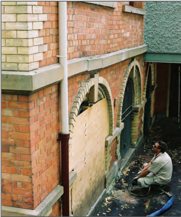
A major section of this heritage-listed school at Darlinghurst, Sydney was re-supported and raised by Uretek prior to effecting masonry repair and replacement.
