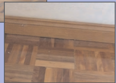
These sets of 'Before' and 'After' photos show how cracks in walls and gaps below skirting boards will usually close up as building footings are lifted. In that case it only remains then for brickwork to be re-pointed and interior wall cracks to be re-plastered.
