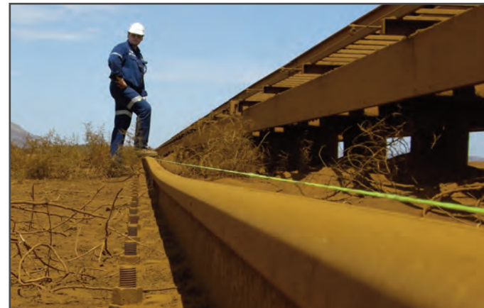
Below: This stacker-reclaimer rail at the West Angelas Mine in The Pilbara Region of WA was also brought back to level and re-supported; allowing the machine to access the vast quantities of stockpiled iron ore again in safety.
