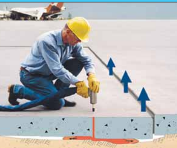
Multi-component, structural resin is injected. It expands immediately, filling any voids and compacting the substrate.
