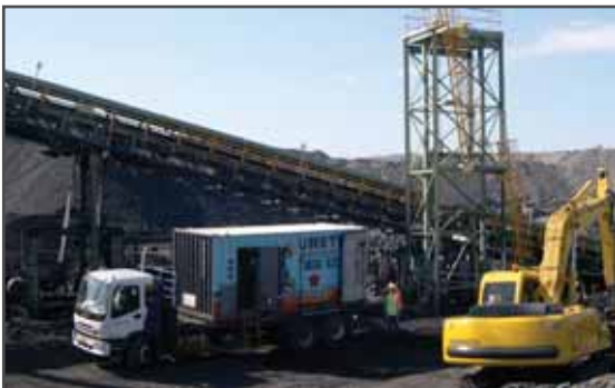
This counter-weight tower base, below, was re-levelled by URETEK.
