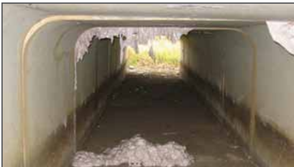
Injected from the roadway above, URETEK resins emerge into the culvert showing sealing is complete.
