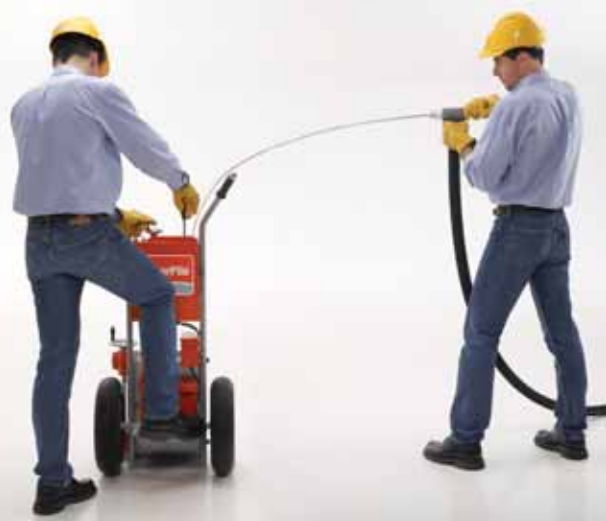
5. Extracting core pipe . . . while injecting resin
