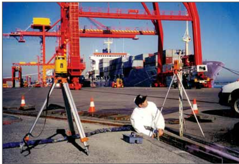
URETEK Slab-Lifting monitored by laser. The area is useable just 30 minutes later!
