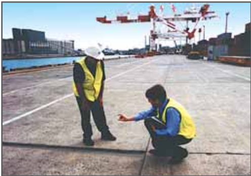
Dockside slab down 50mm.
