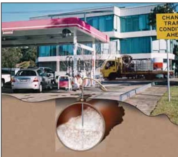
Injected from the roadway above, URETEK resins emerge into the culvert showing sealing is complete.
