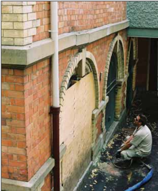
A major section of this heritage-listed school in Darlinghurst, Sydney, was re-supported and raised by URETEK prior to effecting masonry repair and replacement.
