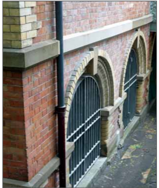
A major section of this heritage-listed school in Darlinghurst, Sydney, was re-supported and raised by URETEK prior to effecting masonry repair and replacement.
