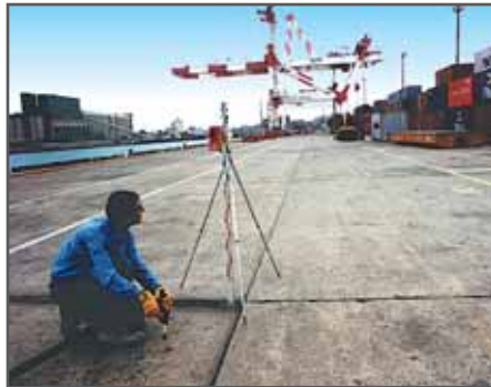
URETEK Slab-Lifting monitored by laser. The area is useable just 30 minutes later!
