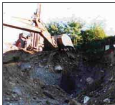
Field testing revealing Deep-Injected URETEK material agglomerating with the ground.
