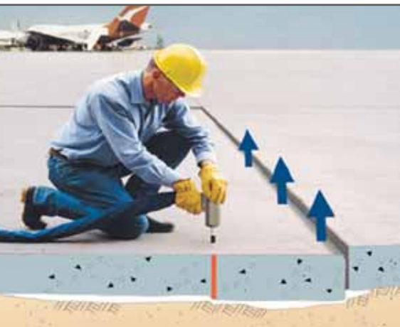
Small holes are drilled through the slab.
