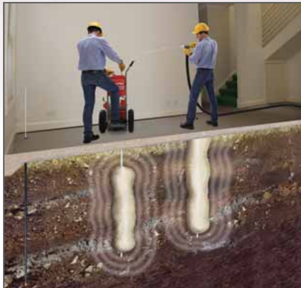
5. Extracting core pipe . . . while injecting resin
